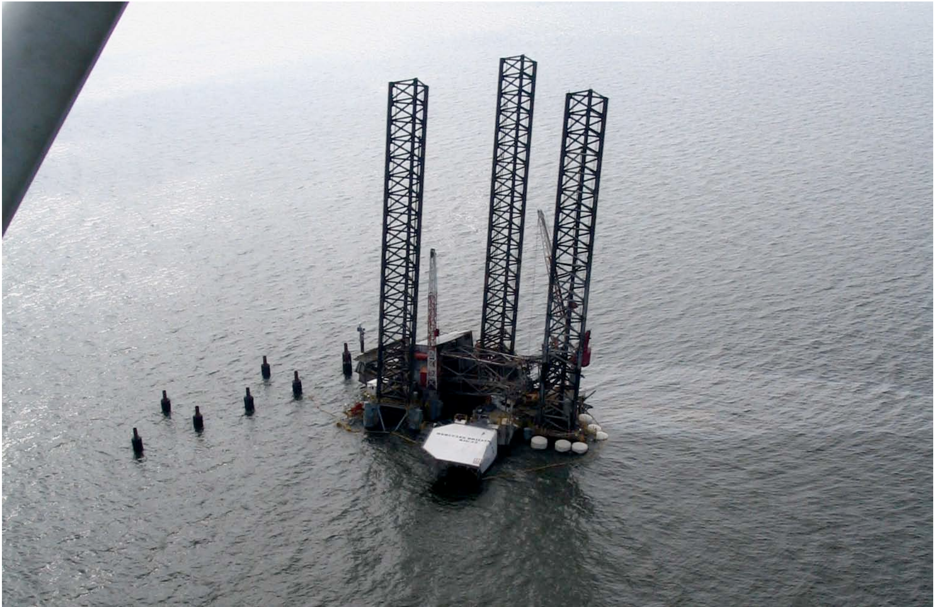
Damaged platform near Breton Island - September 30, 2005. (It really is leaning)
